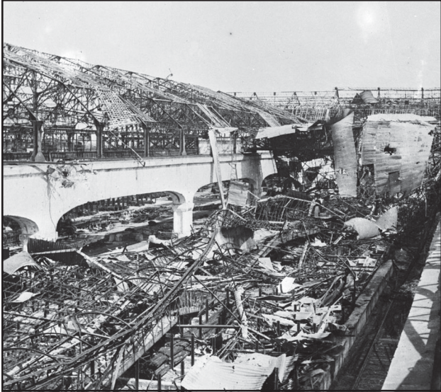
French Steel Plant, 1945
