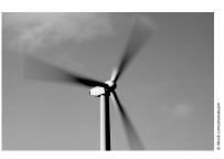
move to face the direction of the wind. The blade speed is set by the force of the wind. A rod attached to the blades turns a motor that changes the power of the wind into electricity. Then the electricity travels hundreds of miles through transmission lines. Homes in large cities, including Houston, Austin, and Dallas, use most of the electricity from the wind farms.
