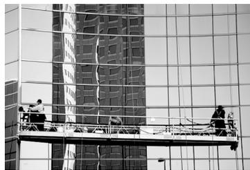
To do their job, skyscraper window washers needed new equipment. The Otis Elevator Company designed the first scaffold for skyscraper window washers. A scaffold is a platform that can be raised and lowered by cables attached to a machine on top of a building. Once the workers are finished, the machine on top of the building lowers them to the next level of windows below.
