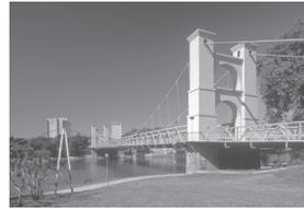
More than 2.7 million bricks were used to build the two double towers at each end of the bridge. Cables attached to the towers supported the wooden roadway over the river. The road was wide enough for two stagecoaches to pass. The bridge was the longest single-span bridge west of the Mississippi River.
