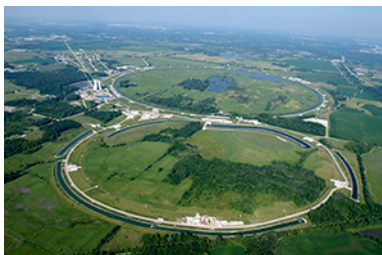
Figure 23.12 The Fermi National Accelerator Laboratory, near Batavia, Illinois, was a subatomic particle collider that accelerated protons and antiprotons to attain energies up to 1 Tev (a trillion electronvolts). The circular ponds near the rings were built to dissipate waste heat. This accelerator was shut down in September 2011. (credit: Fermilab, Reidar Hahn)
