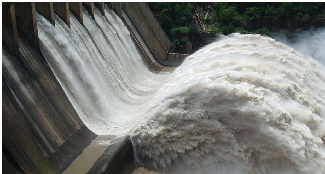
Figure 19.1 Electric energy in massive quantities is transmitted from this hydroelectric facility, the Srisailem power station located along the Krishna River in India, by the movement of charge—that is, by electric current. (credit: Chintohere, Wikimedia Commons)
