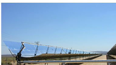
Figure 16.13 Parabolic trough collectors are used to generate electricity in southern California. (credit: kjkolb, Wikimedia Commons)
