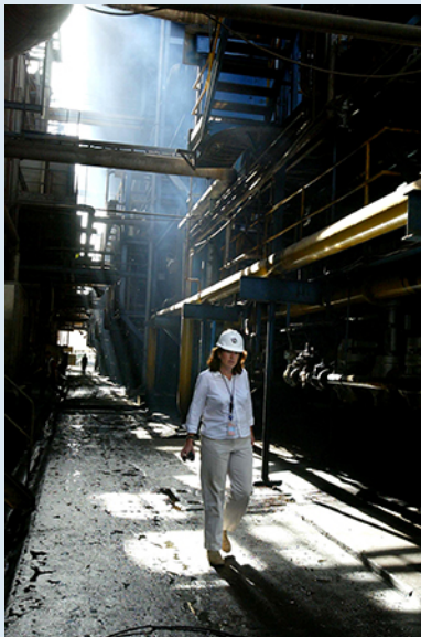
Figure 12.2 An engineer makes a site visit to the Baghdad South power plant.
