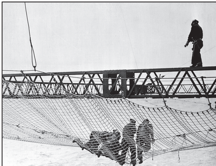
A Golden Gate Bridge innovation, a safety net, was rigged to catch workers if they fell during deck construction.
