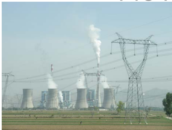
Figure 7.26 Tremendous amounts of electric power are generated by coal-fired power plants such as this one in China, but an even larger amount of power goes into heat transfer to the surroundings. The large cooling towers here are needed to transfer heat as rapidly as it is produced. The transfer of heat is not unique to coal plants but is an unavoidable consequence of generating electric power from any fuel—nuclear, coal, oil, natural gas, or the like. (credit: Kleinolive, Wikimedia Commons)
